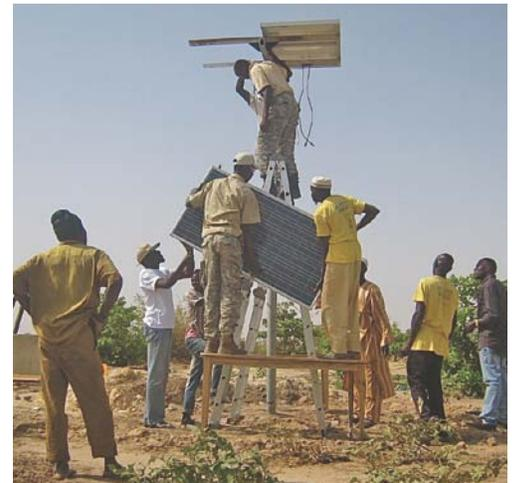
**CREATE! team and community members installing the solar array for the new well and pump in Fass Koffe.**
