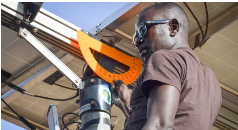
Driver and Field Assistant Pape Ba is attentive to the maintenance of the solar arrays that power water pumping in all thirteen of CREATE!'s partner communities. He adjusts the tilt angle of the panels to maximize the solar energy harvested from the sun.
